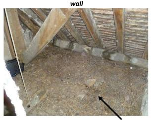
Fig. 4. Hole in the loft floor, largely concealed by detritus
